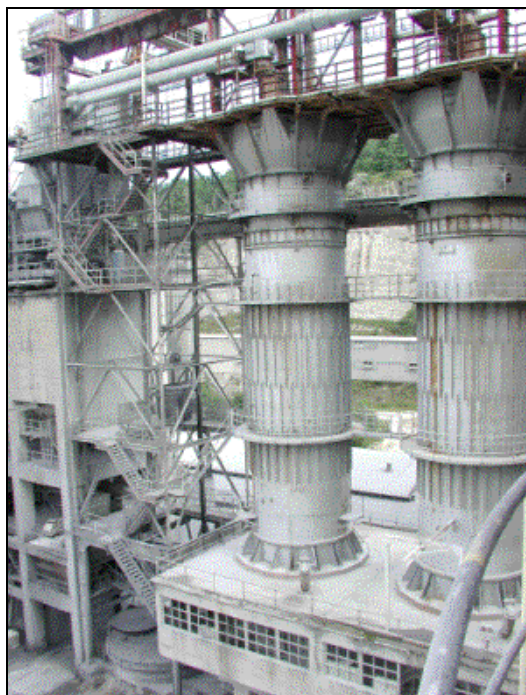
Figure 2.21: Mixed feed shaft kiln [44, EuLA, 2006]
