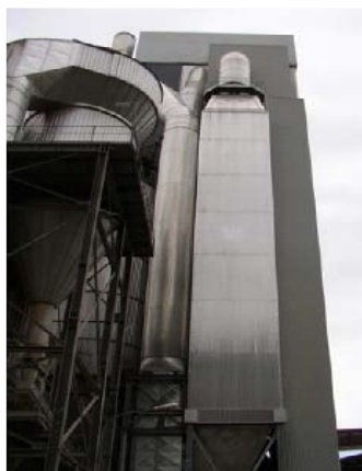
Figure 1.66: Example of an SCR installation [140, Italy, 2007]
